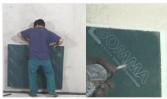
Place the panel on the right wall position and produce 5 holes per panel with the driller (one in the centre and one in the four corners)
