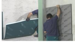
Apply the panel on the wall by forcing with homogeneous pressure.
