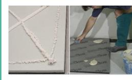
Lay points of a gypsumbased glue on the ground panel or use a low-expansion polyurethane glue
