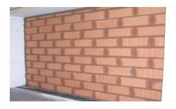
Build up the wall by caring to joint the blocks with mortar on both vertical and horizontal joints.
