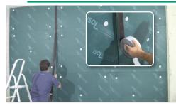
When all panels are fixed seal the panel joints with the "Stik" tape.
