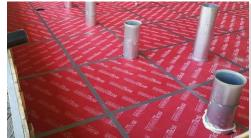
Seal the horizontal and vertical joints carefully with the Stik tape.
