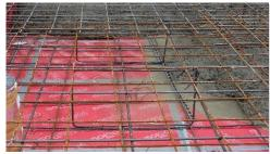
A reinforcement steel mesh should be properly designed and installed depending on the screed dimensions. Build the floating slab directly on the Megapoint layer.
