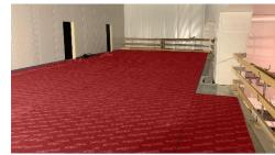
Lay the Megapoint panels taking care of placing them without leaving gaps or cavities along the edges of the joints.
