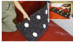
In case of pit, glue the panels Megamat to the walls using Selena Tytan 60s glue.
